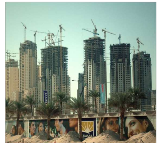
THE OLD, THE NEW
