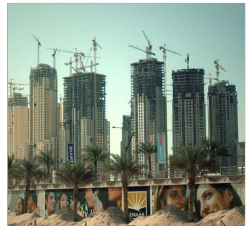
THE OLD, THE NEW
